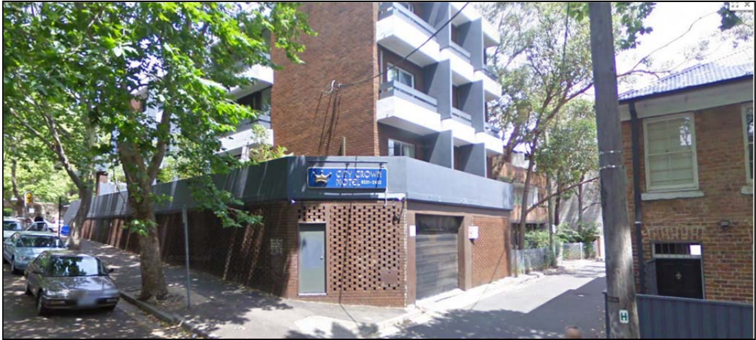
Figure 5: View of existing building at the rear
