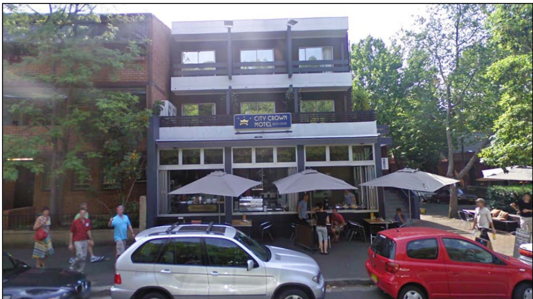
Figure 2: View of existing building from Crown Street
